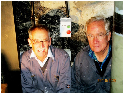
New starter box on wall with Jim and John
