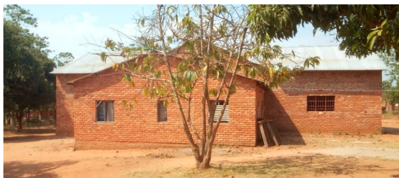
Rear view of church
